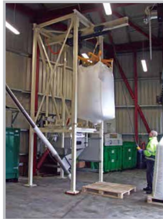
3. Traversing bag into position
